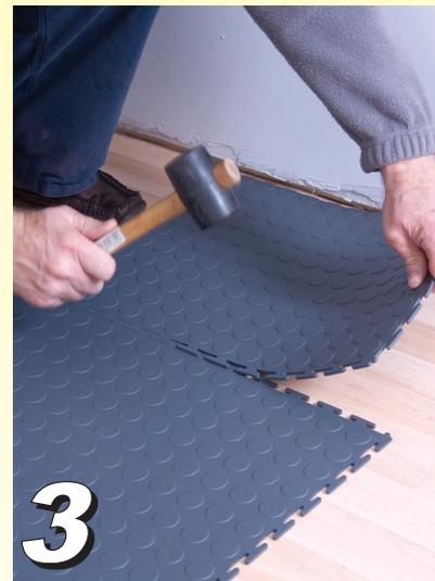
The tiles are designed to fit tightly together. Use a rubber mallet to hammer the tiles into position. On reaching the walls, cut the edge tiles so as to leave 1/4in wide gap between tiles and the wall.
