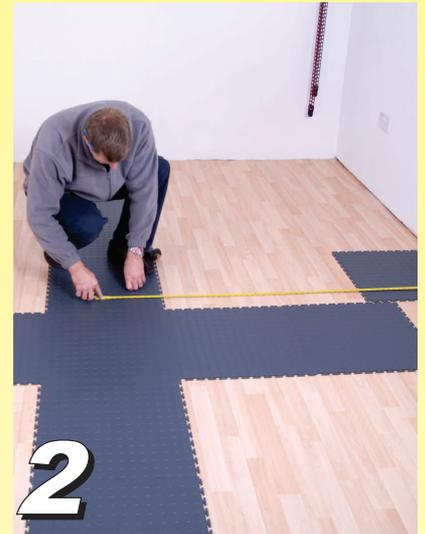
Measure the length and width of the room and divide the dimensions in two. Locate and mark the centre of the room. This is the approximate starting point for the installation. Check the number of full tiles and the width of part tiles required to reach the walls in each direction.
