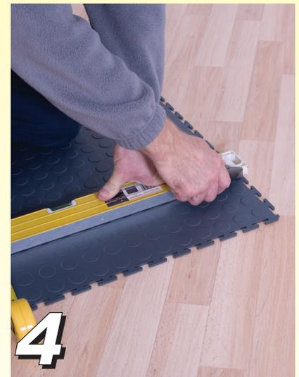
Cutting the edge tiles should be done with a sharp blade. A good non-slip straightedge should be used. It is better to make several light cuts than one heavy cut. Always cut the tile from the front. A cutting board should be used to prevent damage.
